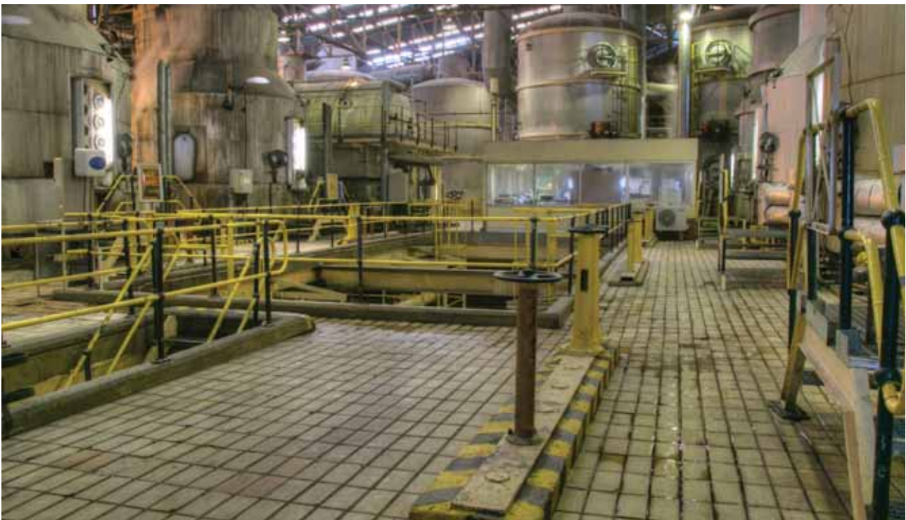
One of the two factories, which collectively crush 741TCHR
