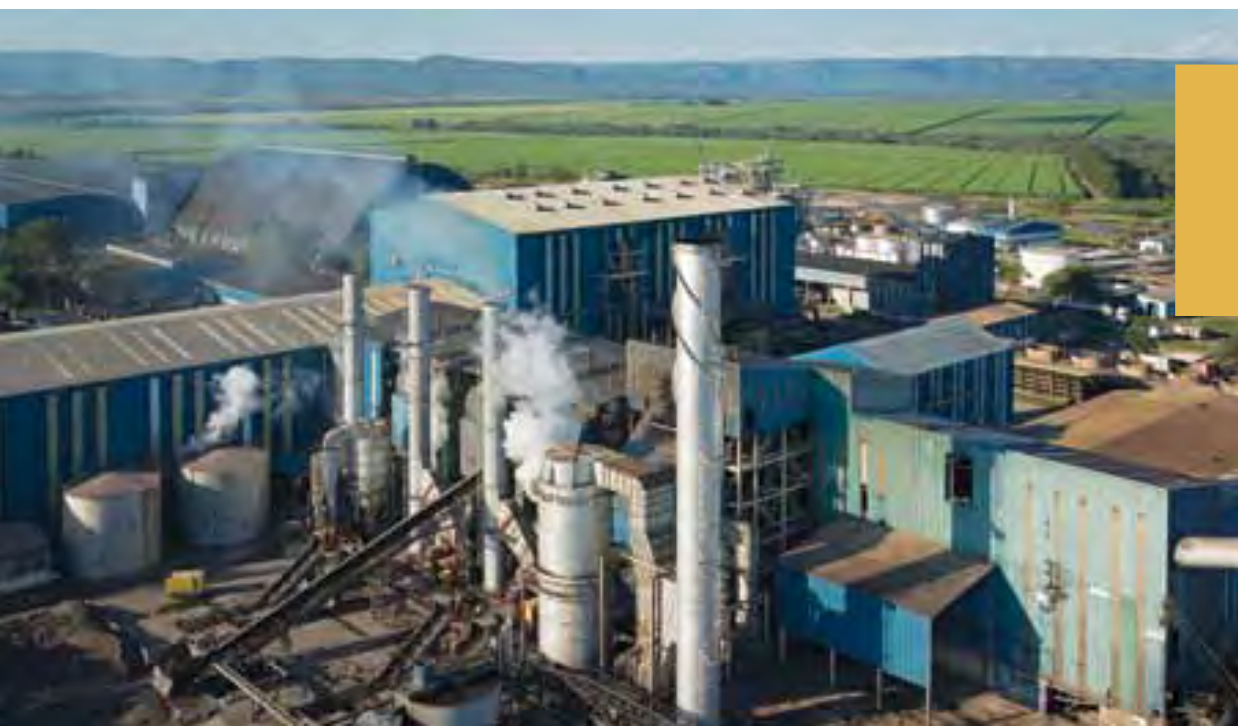
Simunye mill with the sugar warehouse and distillery behind.
