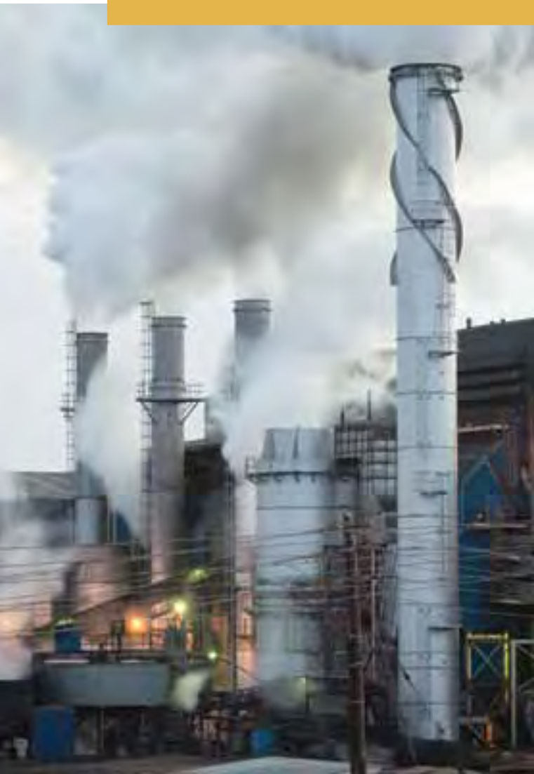
Boiler stacks at Simunye mill.
