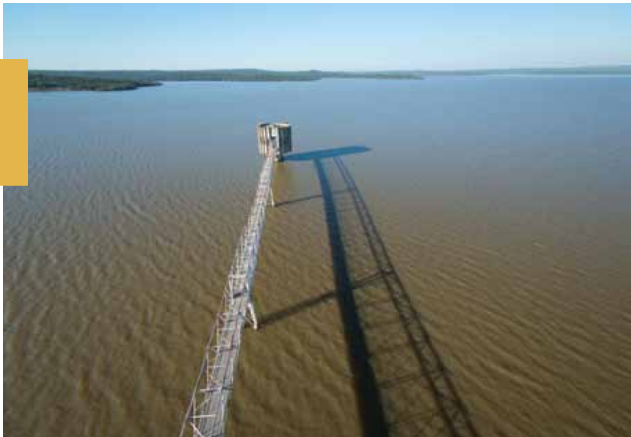
The Mnjoli Dam on the Mbuluzi River - one of our key water sources.
