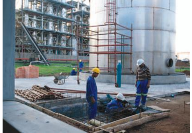
Construction of the Reverse Osmosis plant is underway.
