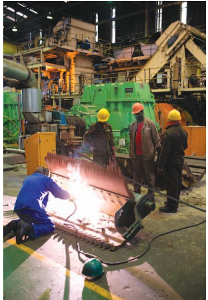
Maintenance being performed at the Simunye plant.
